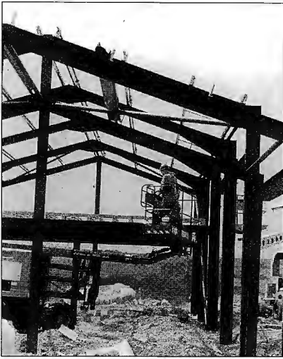
The new workshop under way
