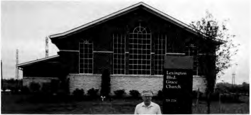
Pastor Drew Garner with the newly built Lexington Boulevard Grace Church in the background – see News
